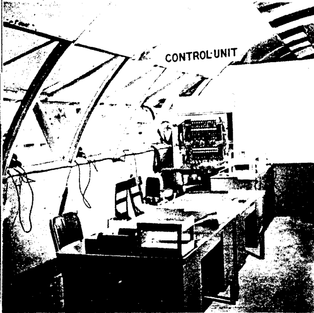
Radio Calls for Maintenance Received Here
